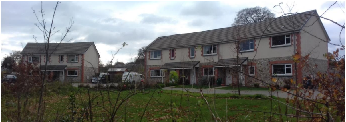
Six affordable homes on a rural exception site in Dalwood, delivered by Corry Valley Community Land Trust
