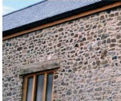
The most characteristic construction material in the Blackdown Hills is chert
