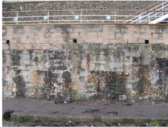
Figure B2: Masonry seawall
