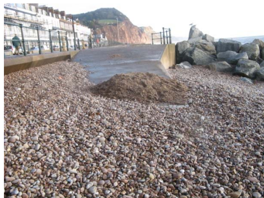
Figure D6: Access ramp
