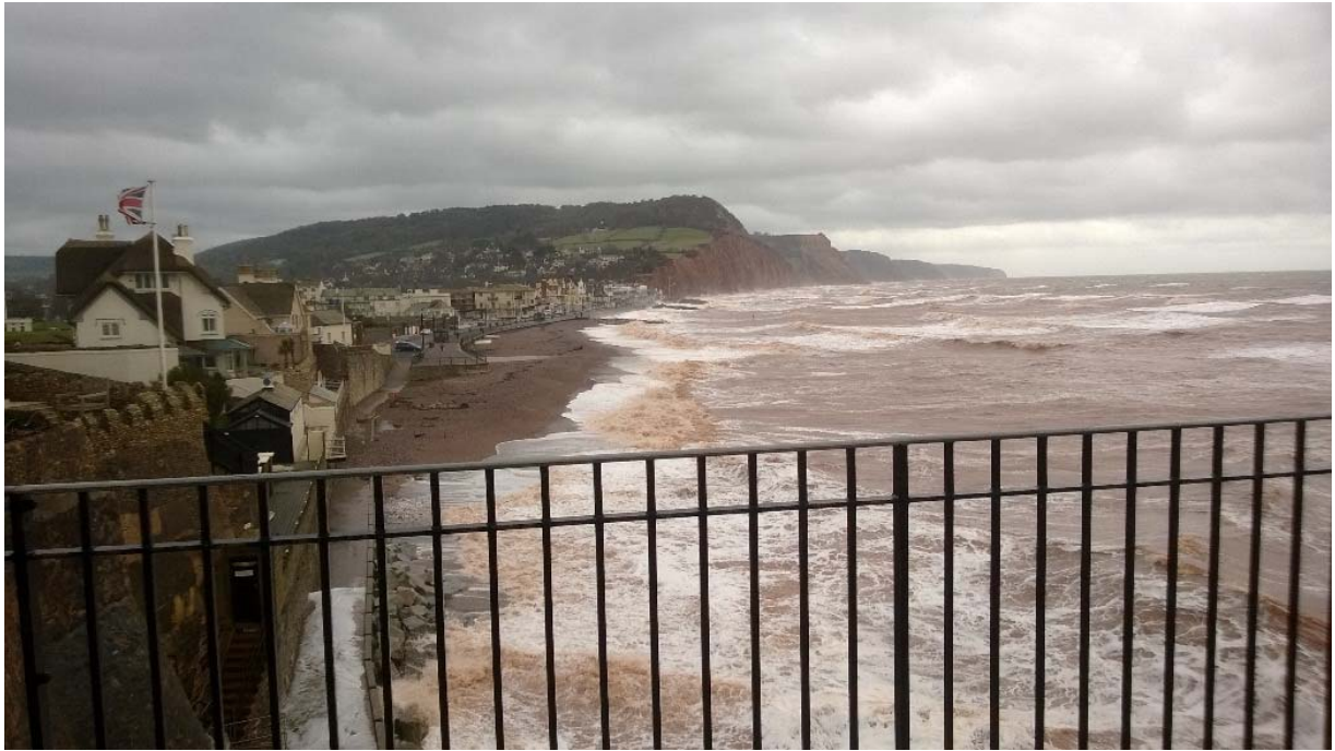
Figure 4-1 Overtopping during February storms of Frontages 2-6
