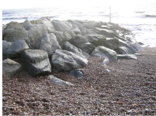
Figure D8: Rock groyne West flank
