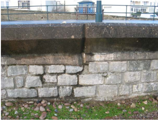
Figure C1: Masonry wall with RC coping
