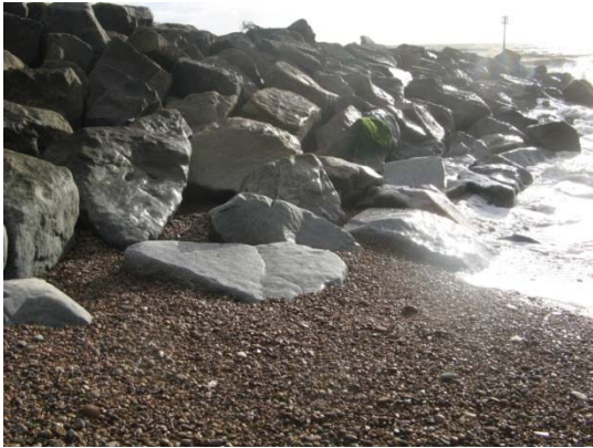
Figure E7: Rock groyne West flank
