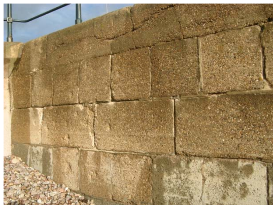
Figure E12: East Pier concrete block joints
