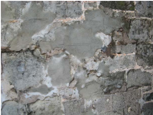
Figure B3: Masonry mortar repairs
