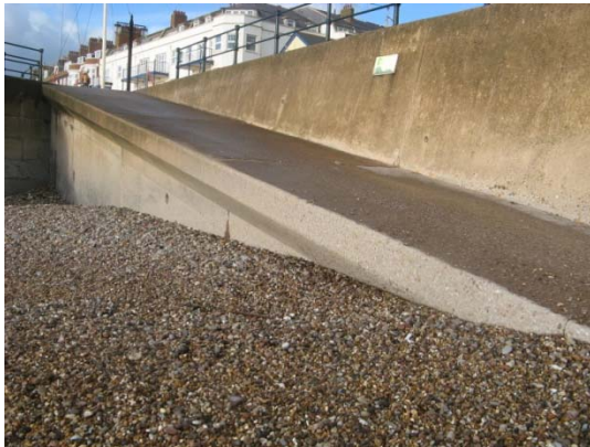
Figure F3: West access ramp
