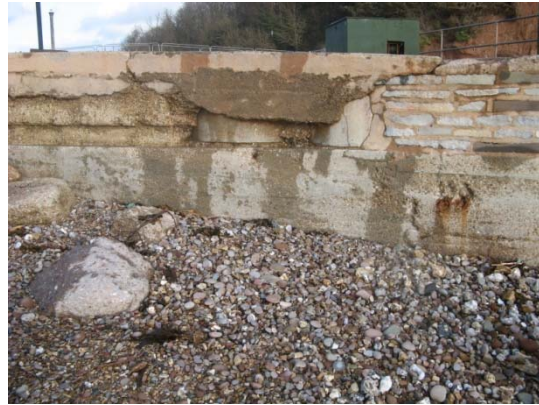
Figure F6: Exposed manhole ring
