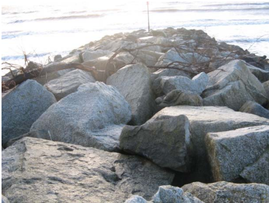
Figure C9: Consistent crest
