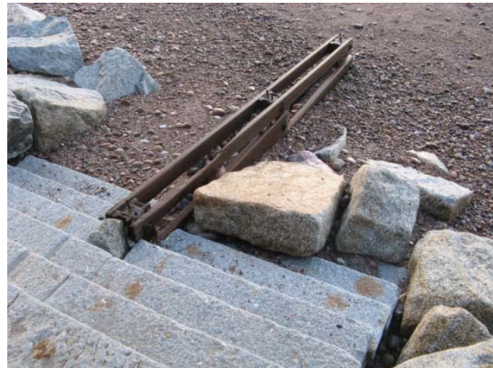
Figure B14: Displaced rocks
