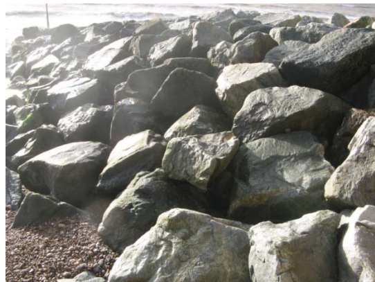
Figure D10: Rock packing and angularity
