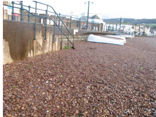
Figure C4: Access stairs and moored boats
