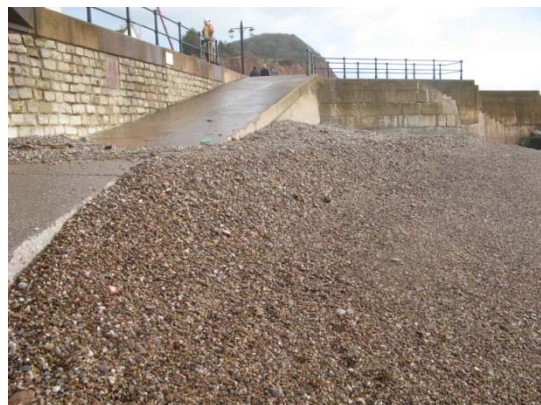
Figure E6: East Pier ramp
