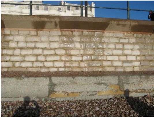
Figure D1: Mortar repairs to apron
