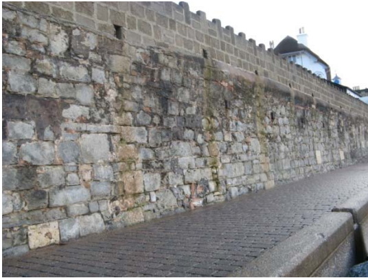
Figure B1: Masonry seawall
