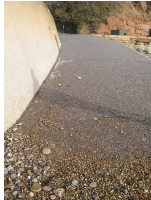
Figure F4: East access ramp
