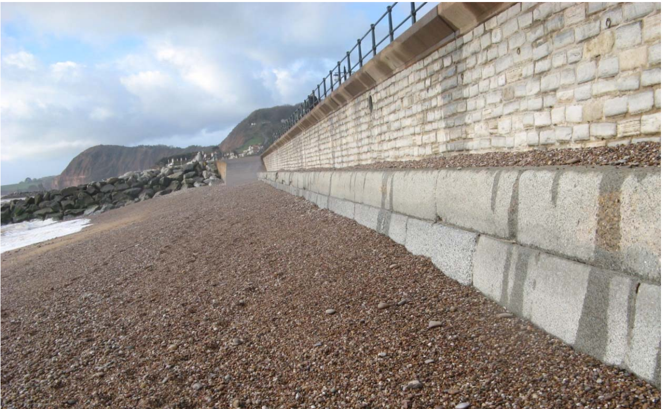
Figure 3-7 Frontage 5 seawall and concrete apron with shingle beach
