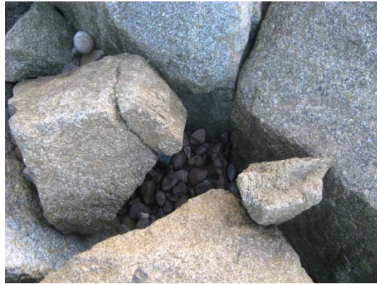
Figure C8: Single infilling and small rocks
