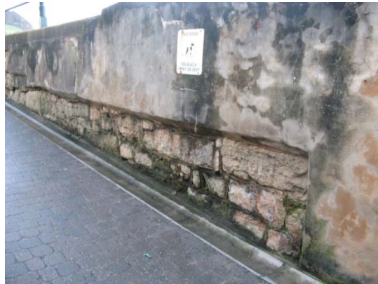
Figure B8: West Pier access ramp
