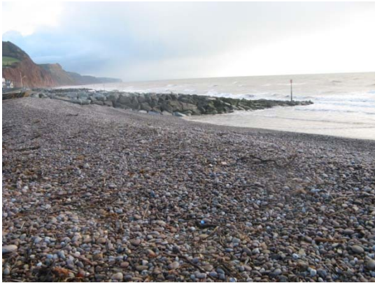
Figure C7: Bedford Steps rock groyne
