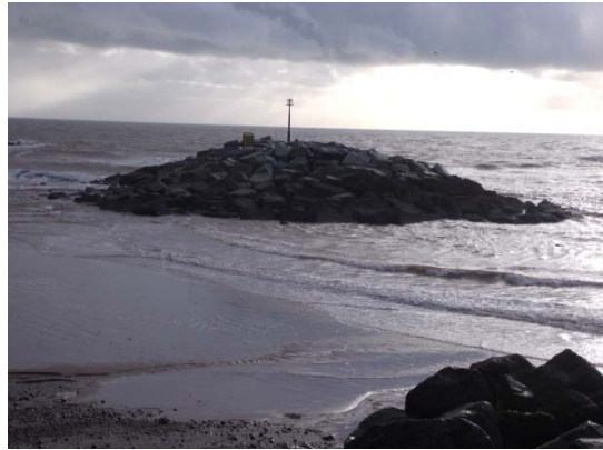
Figure B16: Western breakwater
