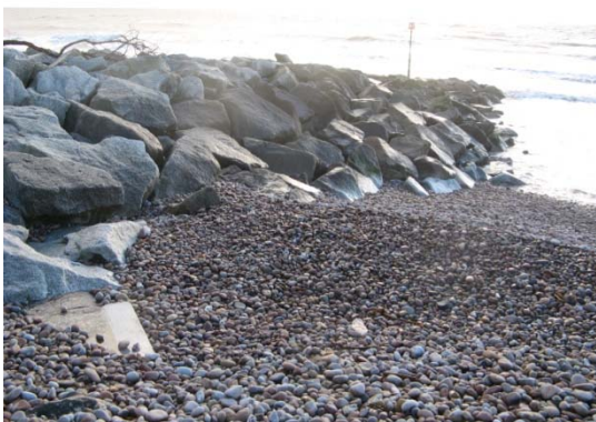
Figure C11: Rock groyne West flank
