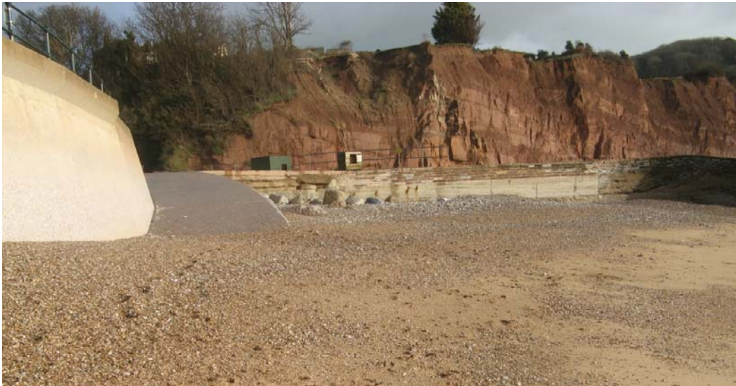
Figure 3-8 Frontage 6 seawall (left) and river training wall (right)
