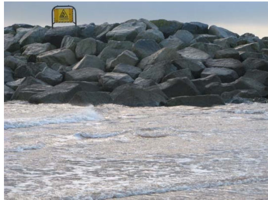
Figure B18: Rock packing on western breakwater
