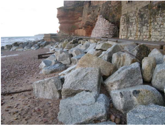
Figure B11: Rock revetment
