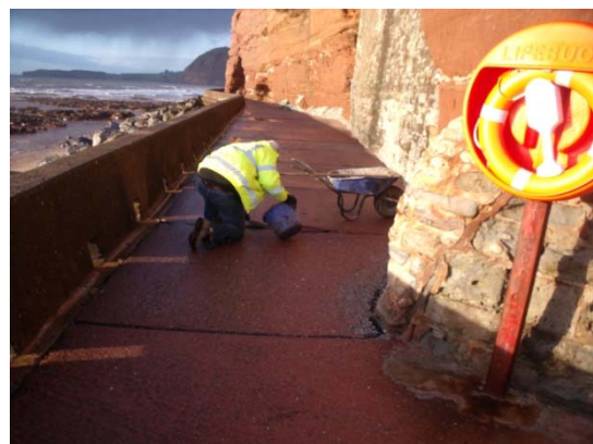
Figure A12: Mortar filling to expansion joints
