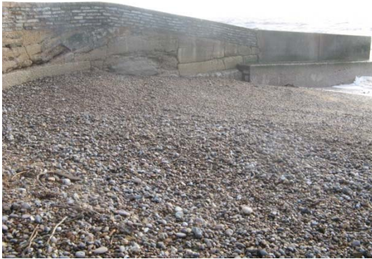
Figure F5: River training wall
