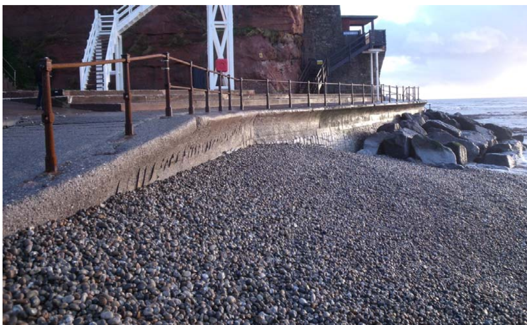
Figure 3-2 Frontage 1 access ramp, seawall and revetment
