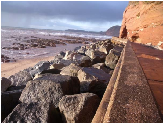
Figure A13: Revetment in front of seawall
