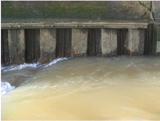
Figure F11: Sheet pile wall
