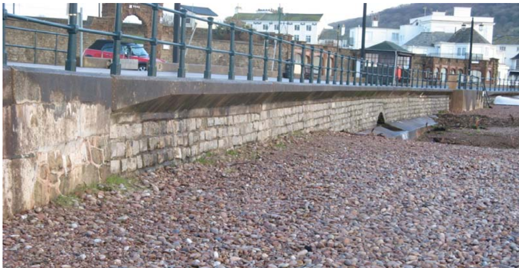
Figure 3-5 Frontage 3 seawall and outfall and a shingle beach
