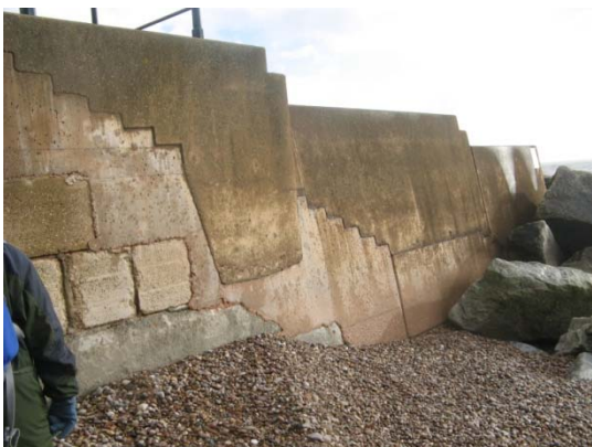
Figure E11: East Pier
