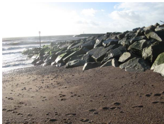
Figure C12: Rock groyne East flank
