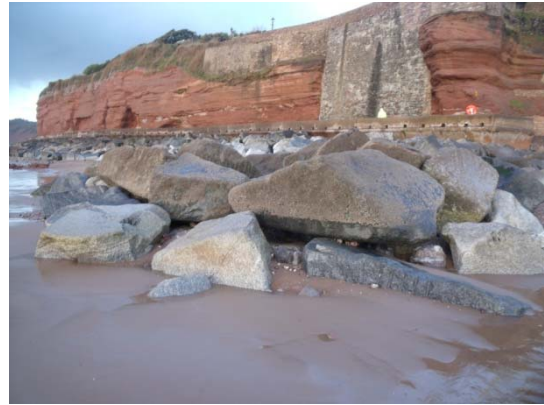
Figure A16: Rock groyne packing and profile
