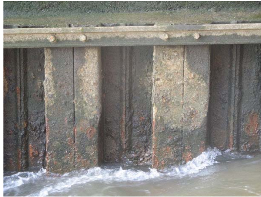
Figure F12: Sheet pile close up
