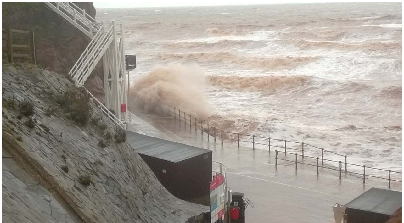
Figure 4-2 Overtopping during February storms of Frontage 1
