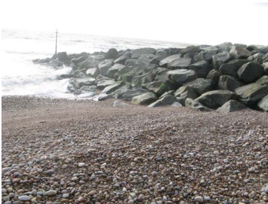
Figure D9: Rock groyne East flank
