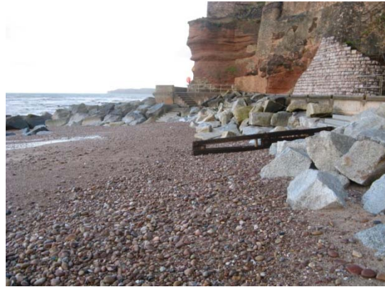
Figure B12: Rock revetment
