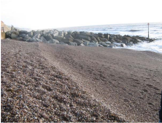
Figure D7: Rock groyne
