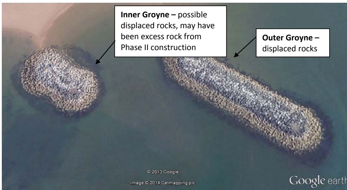
Figure 3-4 Frontage 2 offshore breakwaters showing good plan profile and displaced rocks
