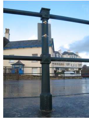
Figure C2: Hand railing free of corrosion
