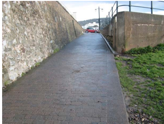
Figure B4: Walkway access ramp
