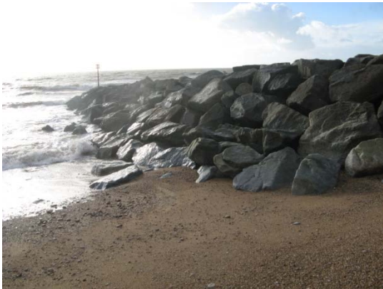
Figure E9: Rock groyne East flank
