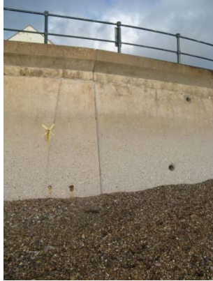
Figure F1: RC faced seawall
