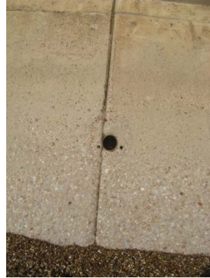
Figure F2: RC wall construction joint
