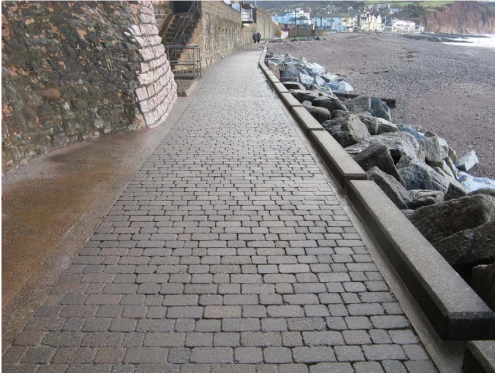
Figure 3-3 Frontage 2 masonry wall, walkway and revetment
