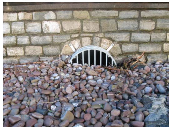
Figure C6: Blocked outfalls
