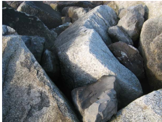
Figure C10: Small rocks used to plug voids
