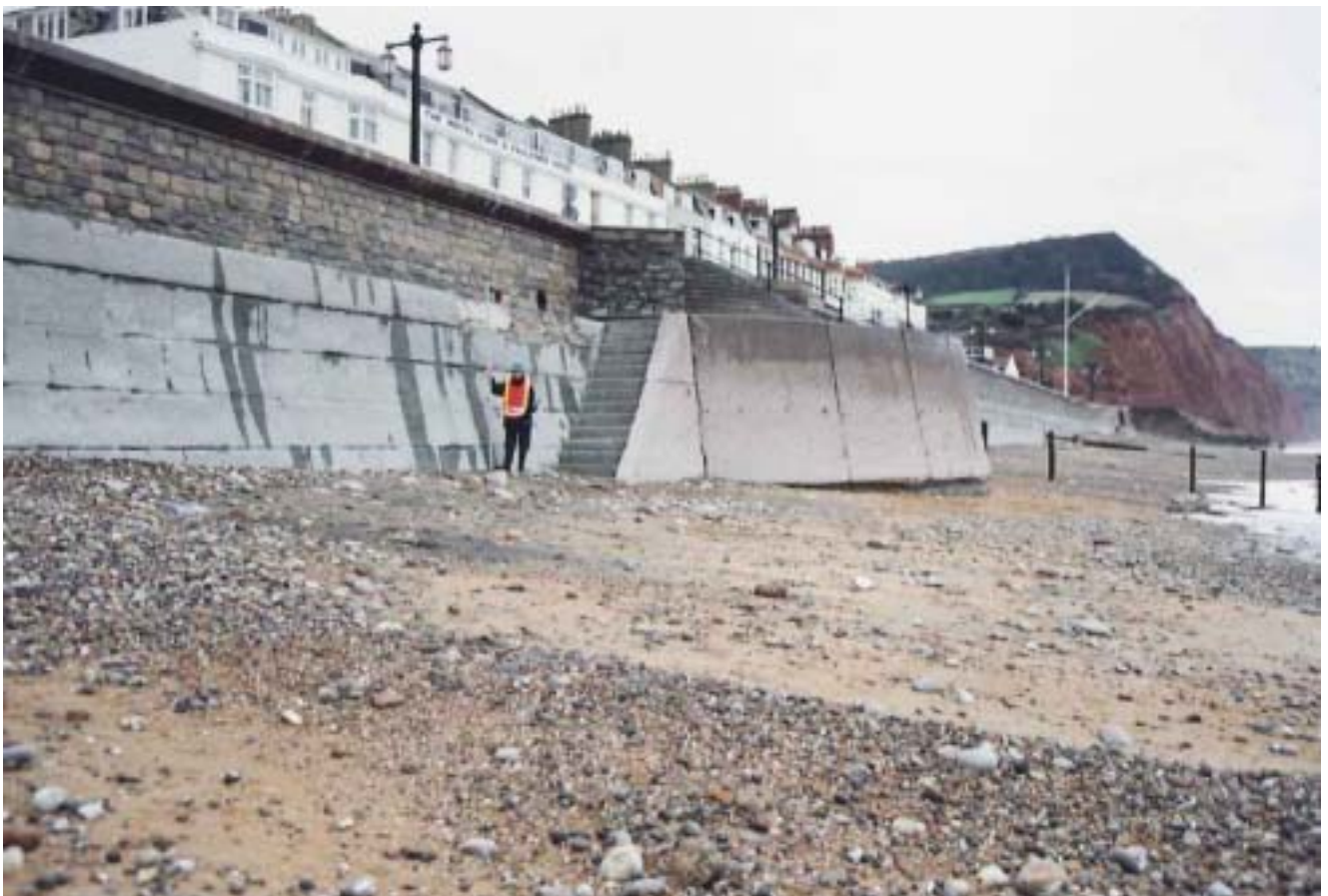
Figure 2-6 January 1993 following beach lowering at Sidmouth (from EDDC records)
