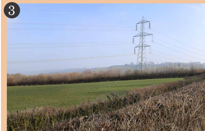
Overhead electric cables run diagonally across the central portion of the site
