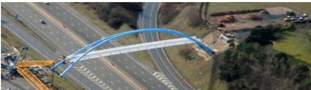
Redhayes bridge spans the M5 providing a link for cyclists and pedestrians
