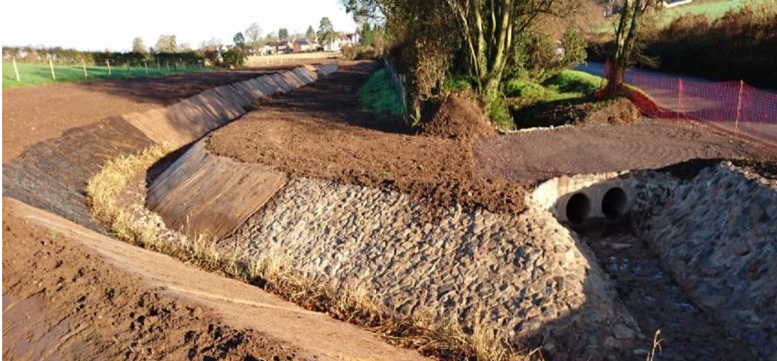
Flood alleviation works at Feniton
