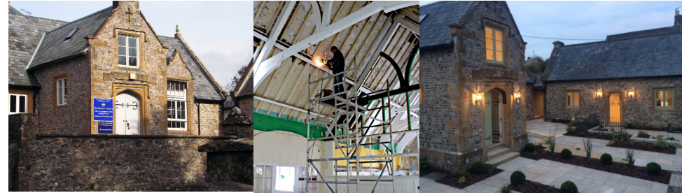
Conversion of the old school building, Chardstock
