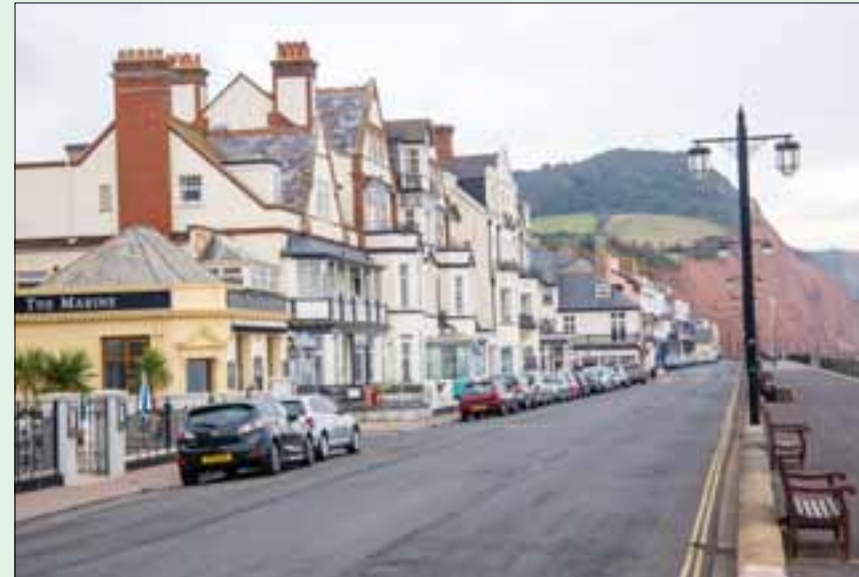
VIEW EAST - ALONG THE ESPLANADE
