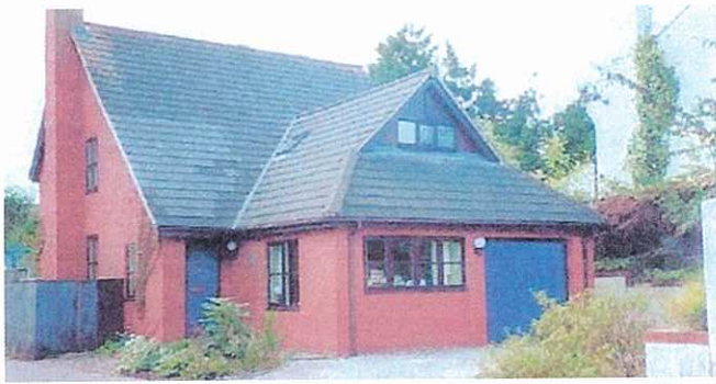
11, Parkhayes – A pleasing pent roof design
