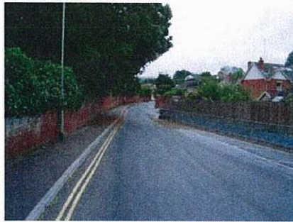
Hind Street showing brick wall
