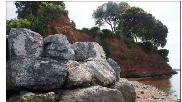
Rock armour protecting eroding headland, Exe Estuary
