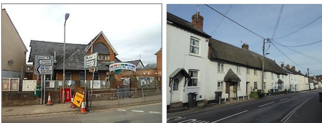
Examples of detracting features in Conservation Areas: Cluttered signage at Ottery St Mary (2013) and overhead power lines at Sidford (2018)
