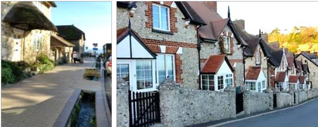
Beer paving - local Beer stone and Beer workers cottages - local flint
