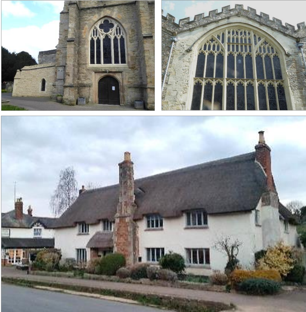
Use of Beer stone at St Giles and St Nicholas parish church, Sidmouth and the Parish Church of St Andrew, Colyton. Renovation with cob and thatch, Otterton
