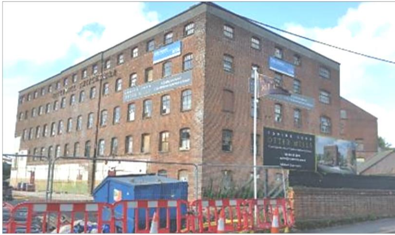
Example: Otter Mill, Switchgear factory and site, Ottery St Mary in 2013 and 2017 (previous page) and 2018 (above)
