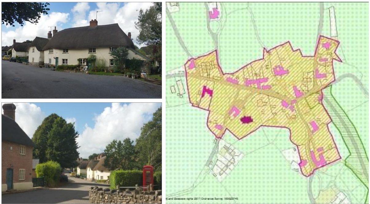
Gittisham village: example of workers cottages and map showing extent of the Conservation Area (yellow) and Listed Buildings (pink).
