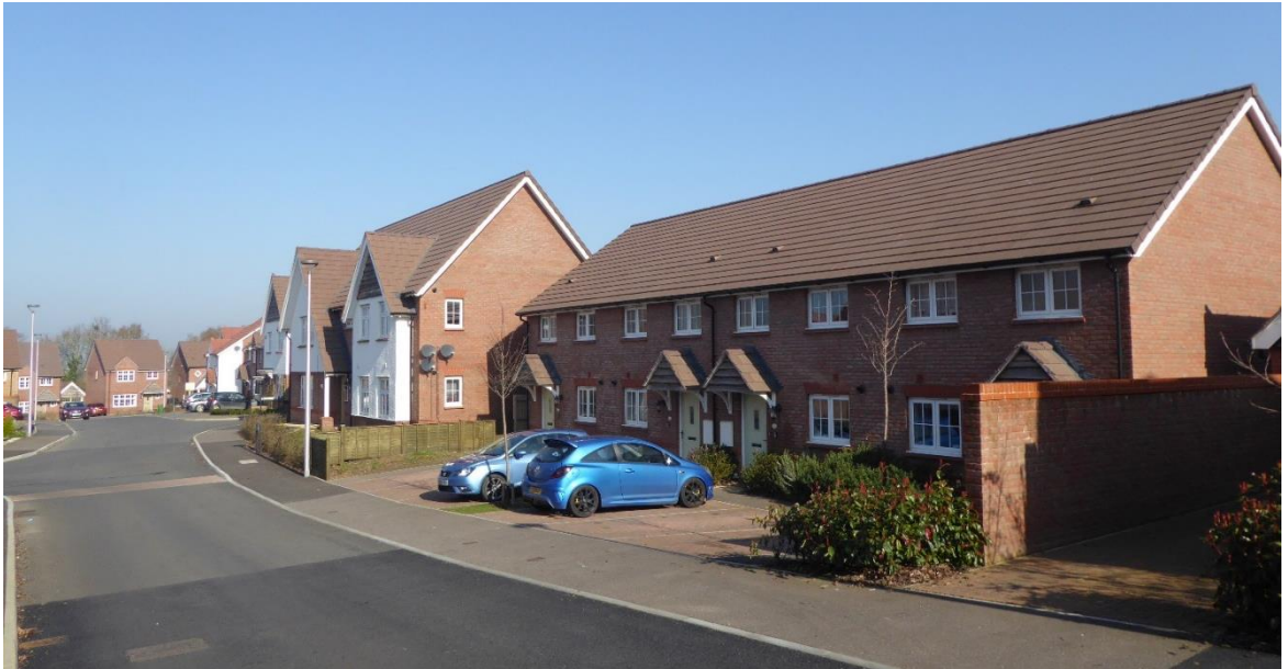
New affordable homes at Ottery St Mary
