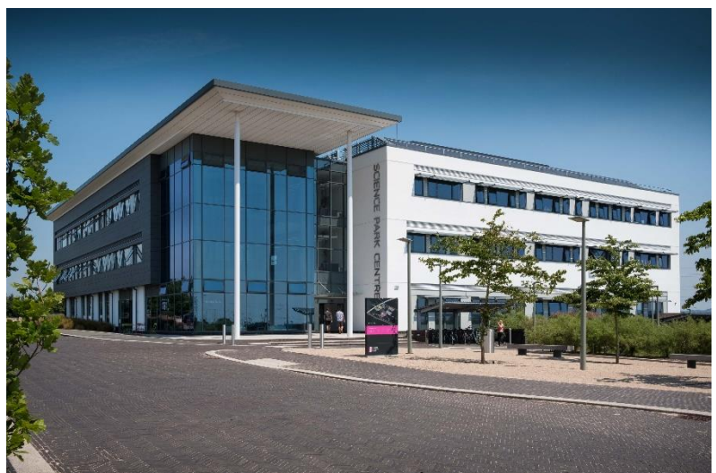
Science park centre in the west end of East Devon
