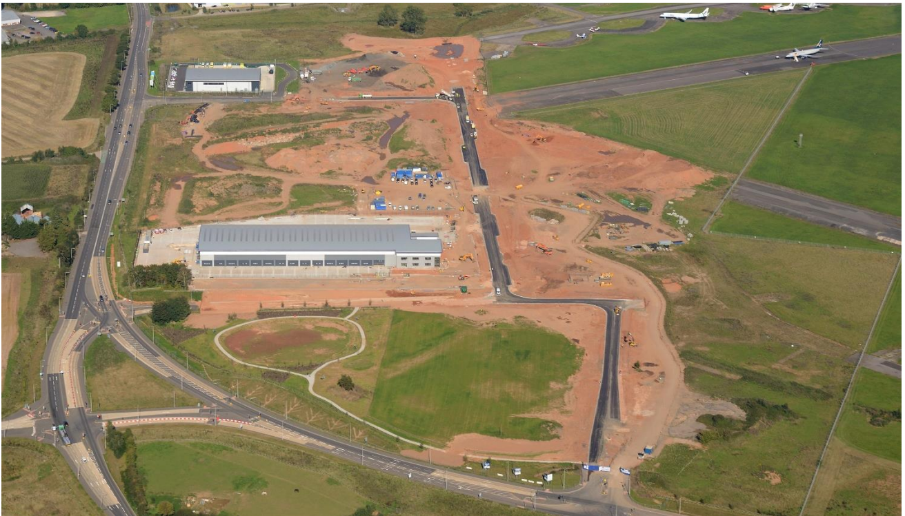
Skypark, next to Exeter Airport, during construction
