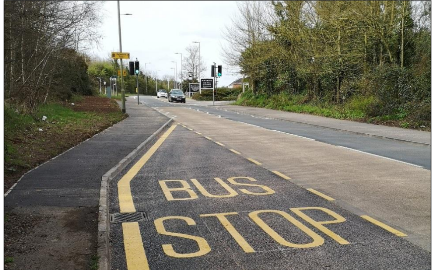
Figure 31 The latest progress towards delivering the Clyst Valley Trail; a crossing at Blackhorse Inn
