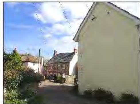
The Hill - an old connecting road to the A35. Lorries struggle to get through the 'dog leg'. Note damage on building
