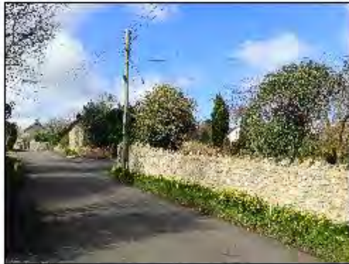
Recently renovated rumble stone wall
