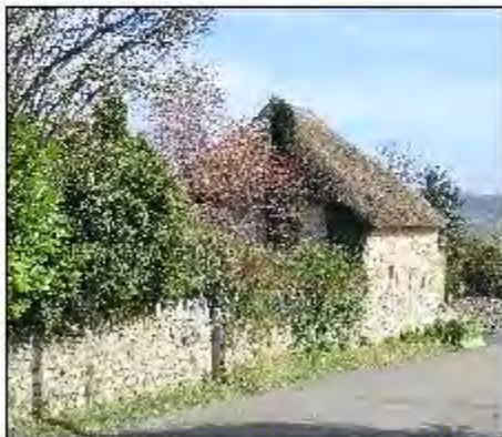
18 th century barn and wall of rumble stone construction
