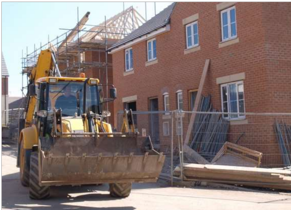
FIGURE 5. Homes under construction.
