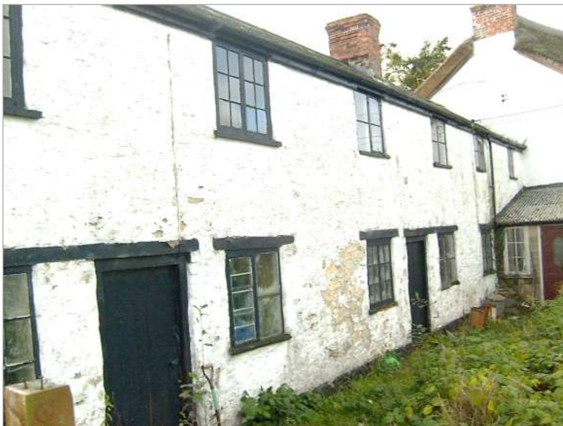
FIGURE 22. Colyford Conservation Area buildings
