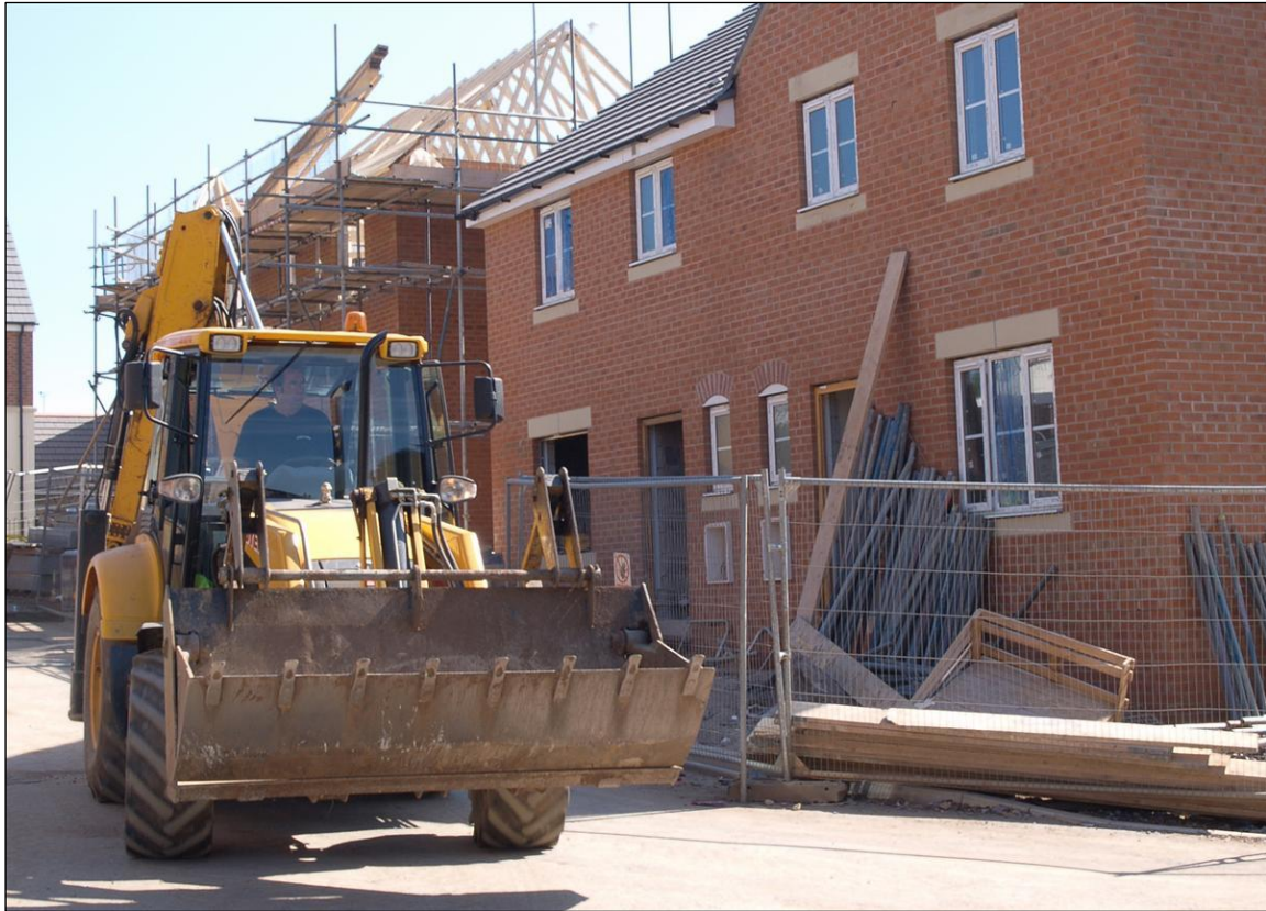
FIGURE 6 Homes under construction
