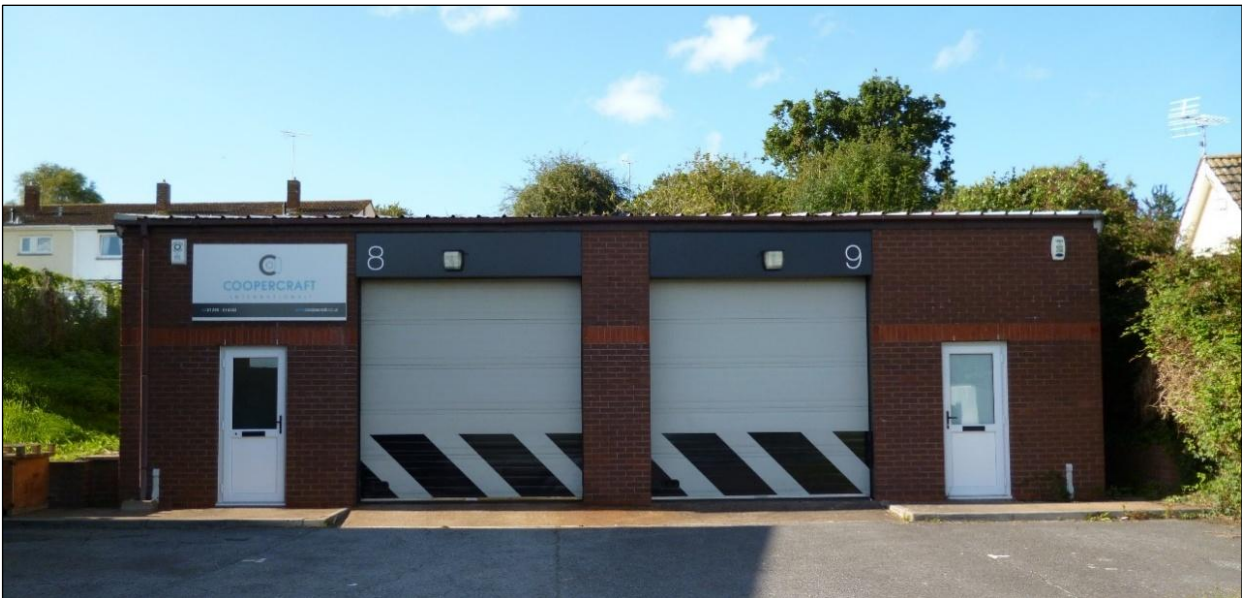
FIGURE 11 Light industrial units
