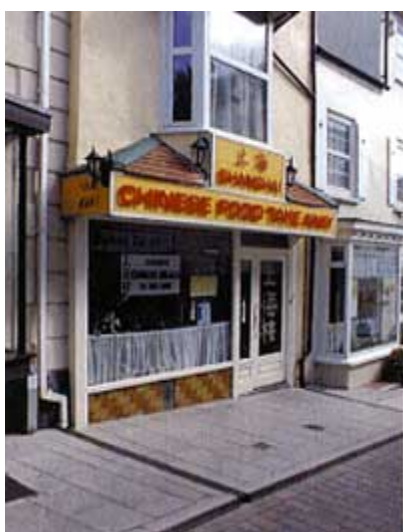
A modern shopfront, respecting tradition and proportions, the tiled roof above the projecting fascia creates a different character
