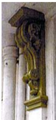
The pilaster and scroll bracket gives framing and strong support to the upper floors
