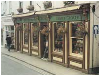
A fine example of a traditional shopfront
