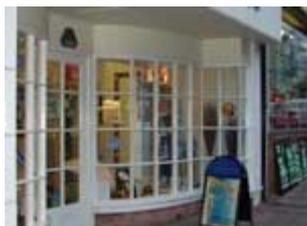
Mullions, normally made of timber, are vertical elements that subdivide panes of glass.
