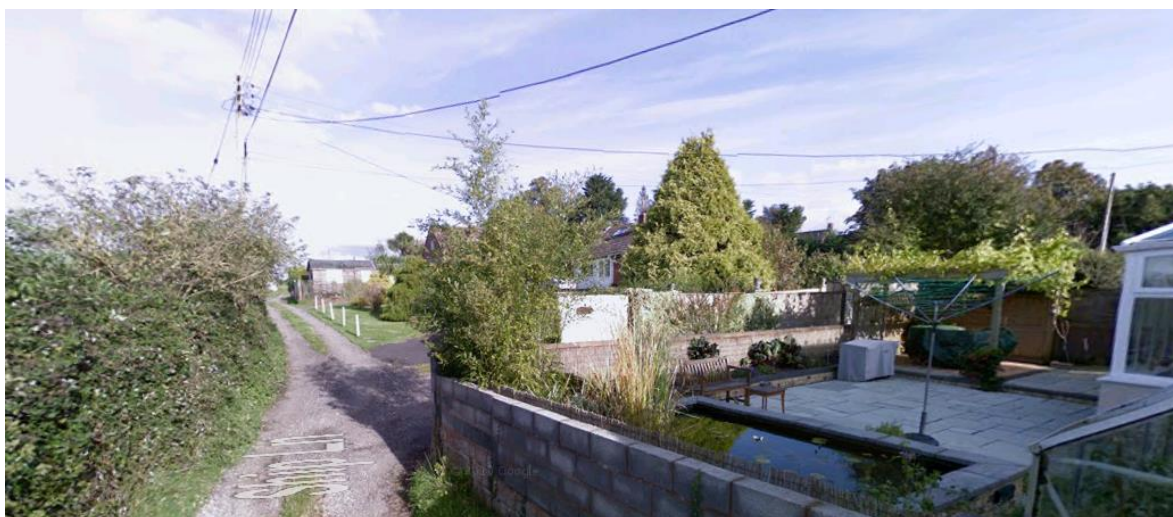
Figure 20: Tightly packed, dense development gives way to more spacious properties and a semi-rural character as you move along Ship Lane
