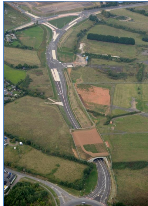
Figure 3: The Clyst Honiton bypass
