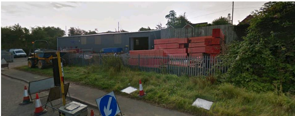
Figure 13: The SW Slating & Tiling site
