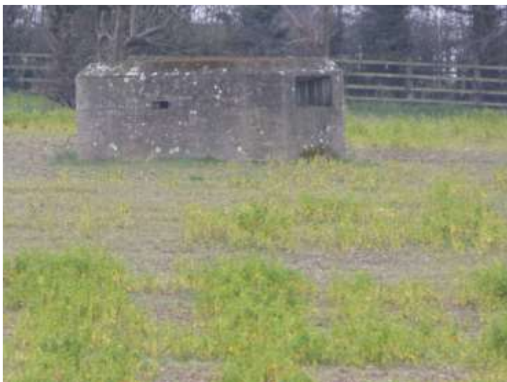
Pill box viewed from public footpath across site.
