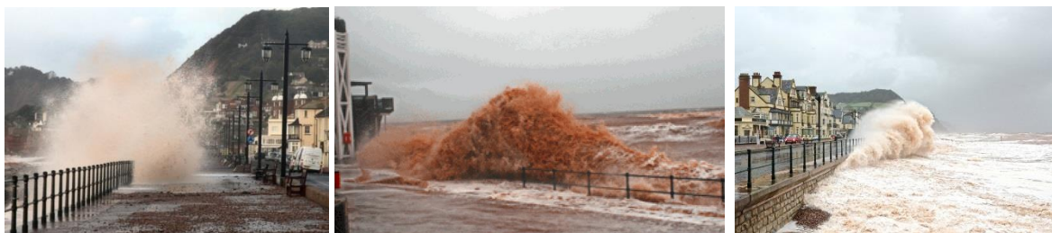
Figure 11.2: Wave Overtopping Along Sidmouth Town
