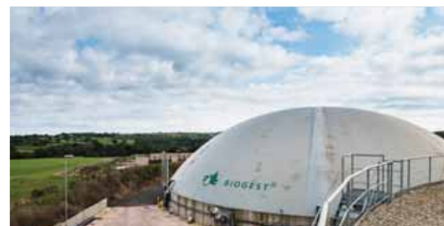
The anaerobic digestion plant at Greendale Farm, a sustainable energy strategy will be delivered
