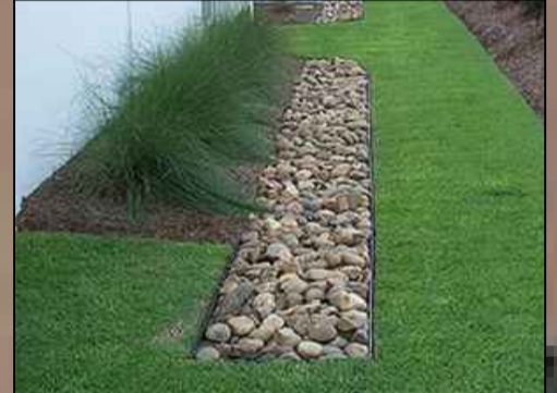
EXAMPLE OF FILTER TRENCH ARRANGEMENT
