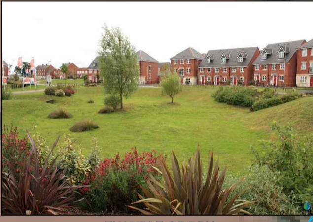
EXAMPLE OF DRY ATTENUATION BASIN
