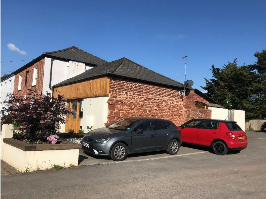
A very good example of render, Heavitree stone and red brick being combined in a new build, which makes a good gateway site along York Terrace
