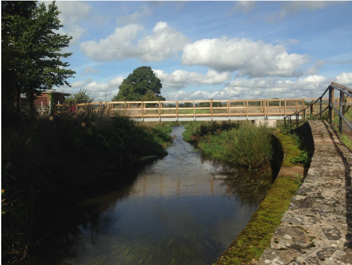
Figure 20 : River Clyst with flood prevention walls and footbridge over.
