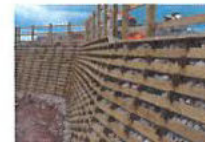
SUPERMARKET: CRIB WALL
