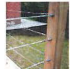
SUPERMARKET: POST AND STRAINED WIRE FENCING
