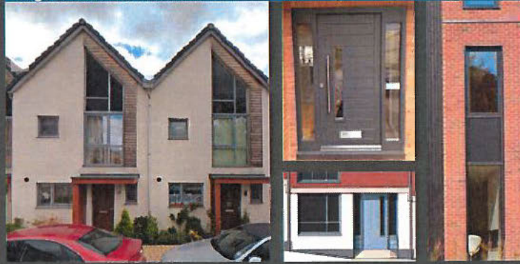
Large Ground Floor Fenestration & Doors to facilitate potential future change of use
