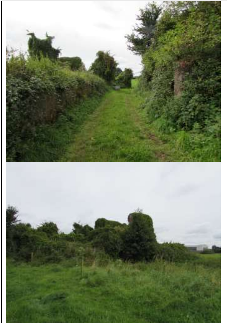
Figure 21: Carrow Mill structures appropriate for part or whole restoration.
