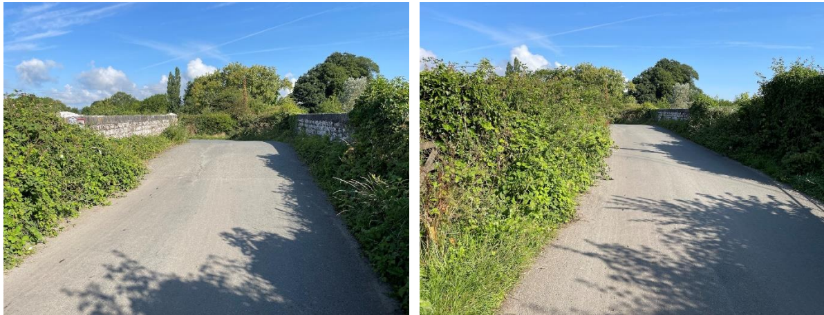
Figure 5: Lilypond Lane Bridge
