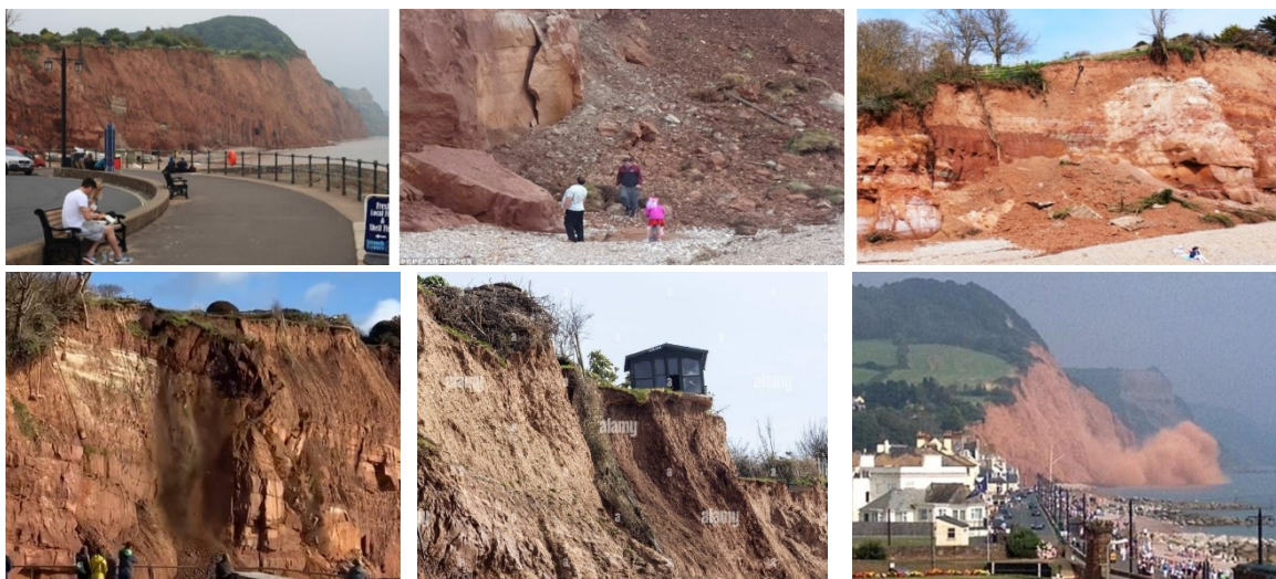
Figure 22: East Beach current arrangement and recent cliff falls
