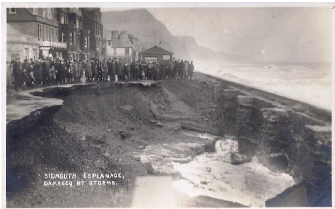
Figure 18: Sidmouth, The Esplanade – Storms damage 1920s
