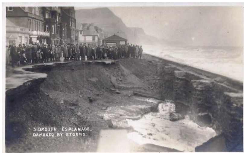
Figure 6: Sidmouth, The Esplanade – Storms damage 1920s
