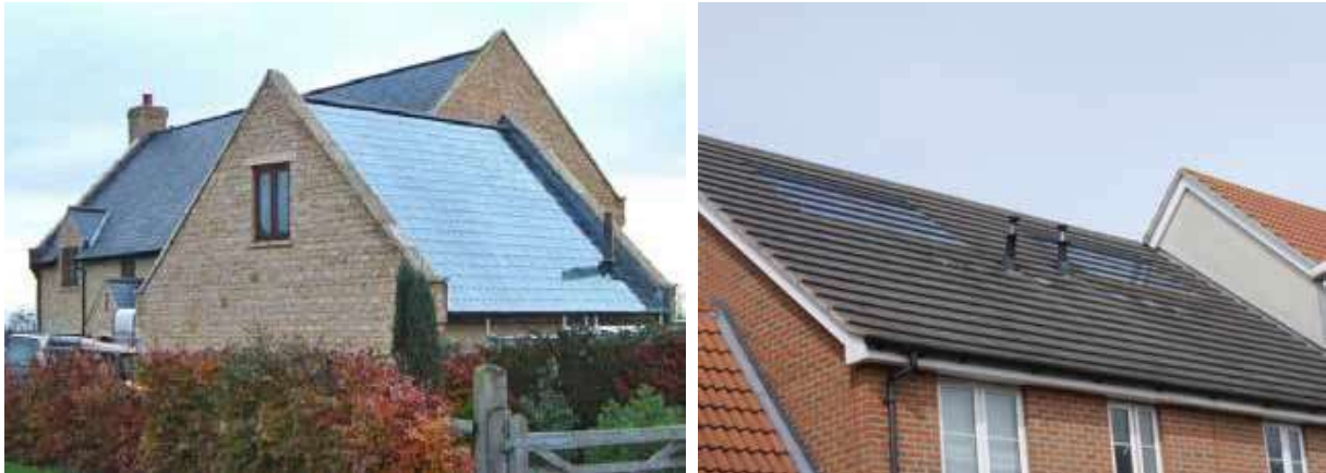
Figure 25: Examples of PV roofing materials now available.
