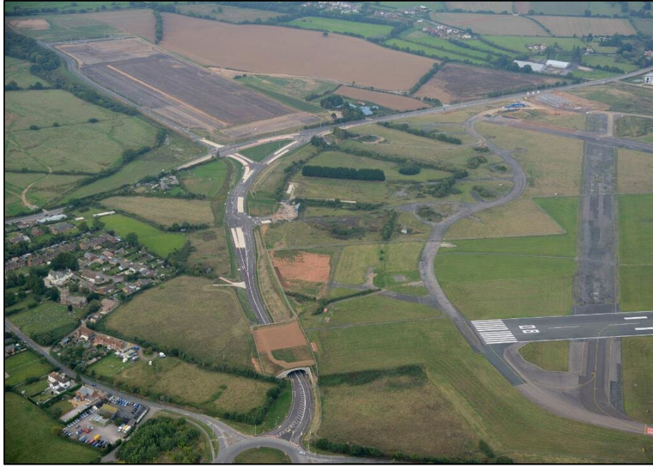
Figure 8: Aerial shot of Clyst Honiton Bypass completed for Cranbrook and Skypark traffic.
