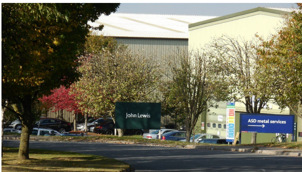
Figure 12: Hill Barton warehouse units.
