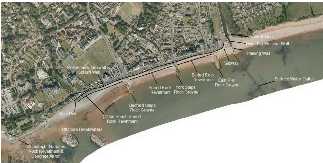
Figure 1-3: Sidmouth's current coastal defence arrangement
