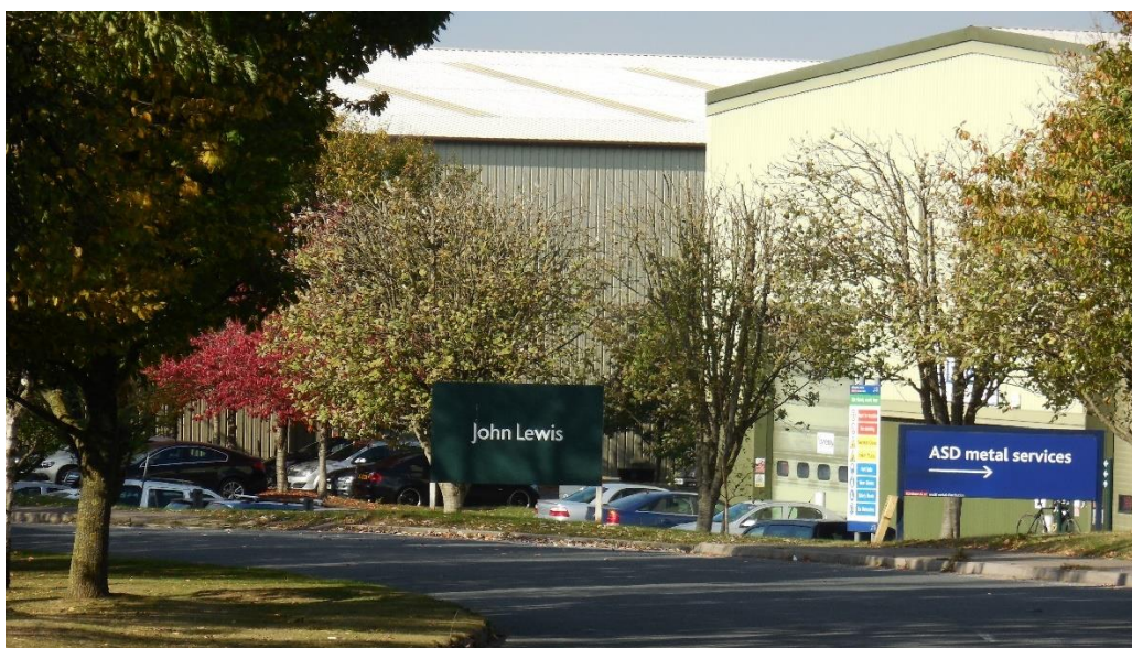
Figure 12: Hill Barton warehouse units.
