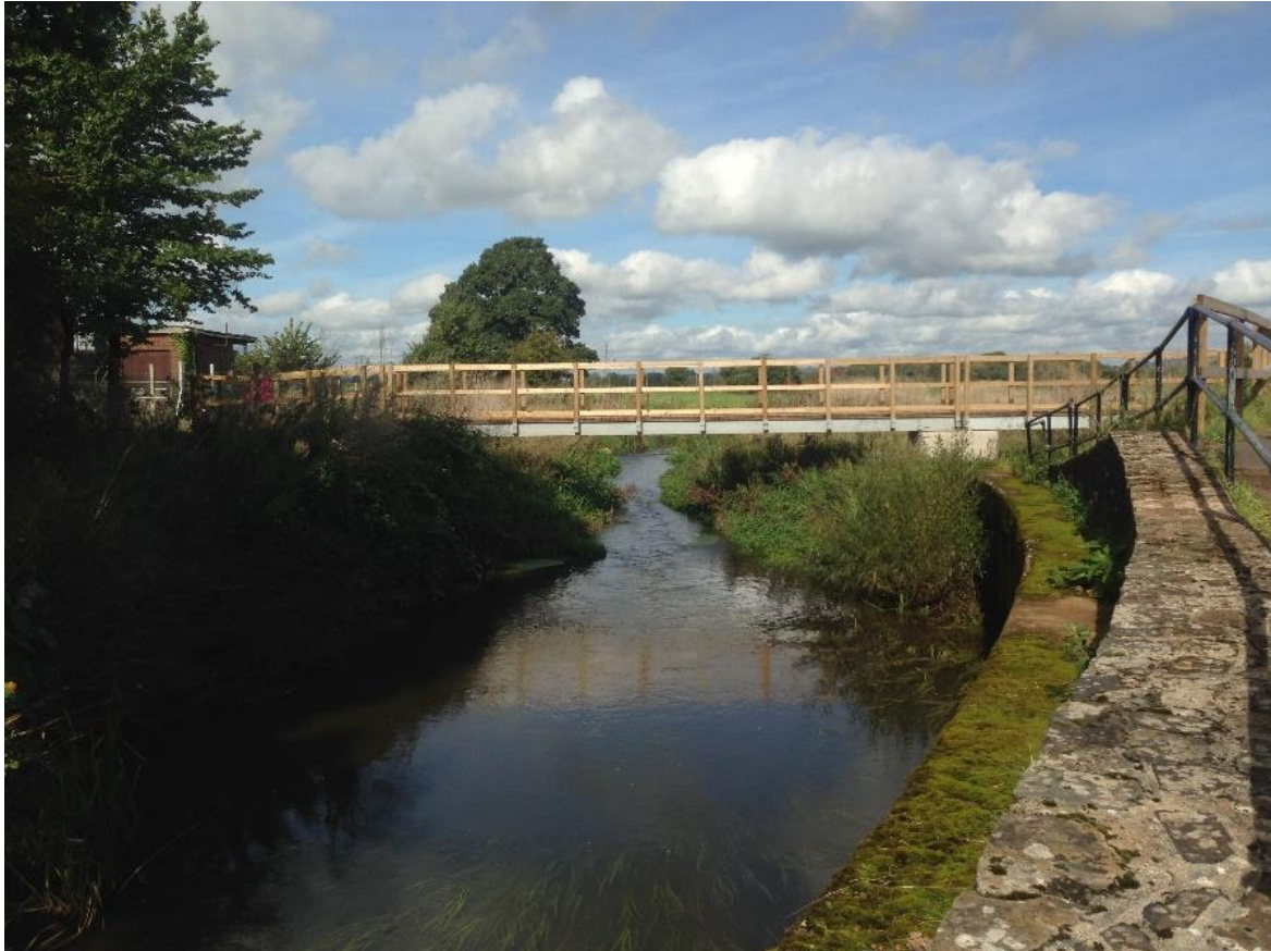
Figure 22 : River Clyst with flood prevention walls and footbridge over.
