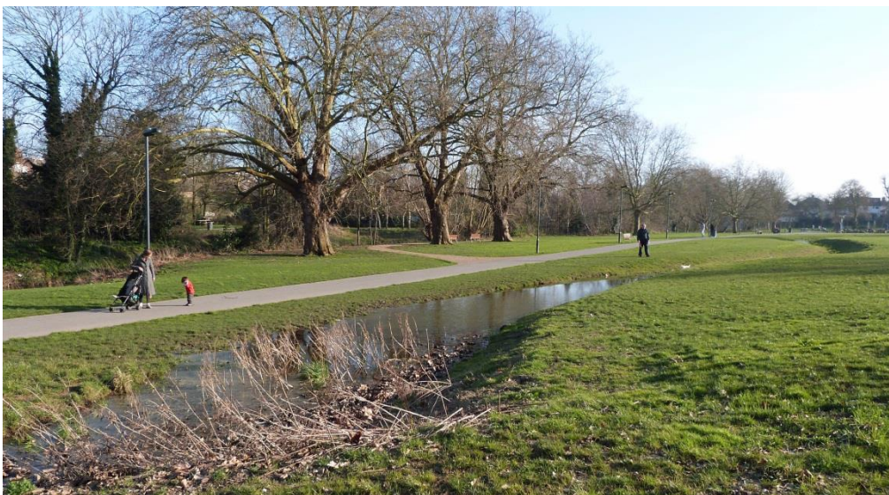
Restored park (and floodplain) in Ladywell Fields, Lewisham with a large swale as part of the landscaping to manage overland flow Source: Peter Bide
