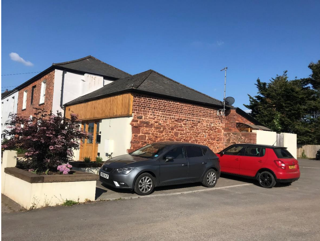
A very good example of render, heavitree stone and red brick being combined in a new build, which makes a good gateway site along York Terrace
