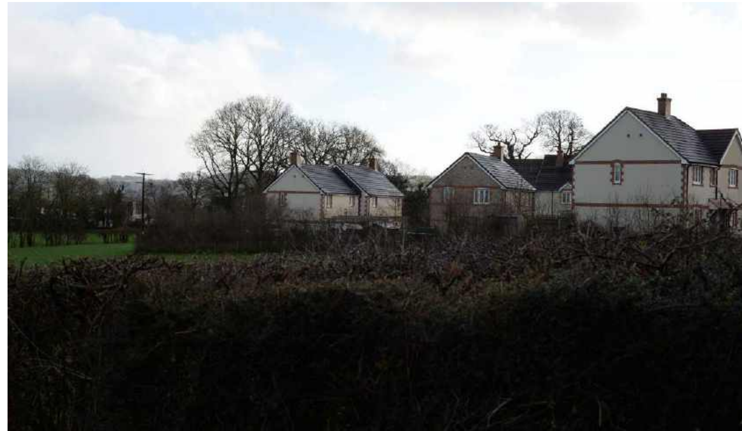
View taken from the A35 looking south towards Dares Field
